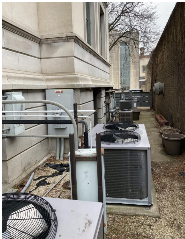
(Equipment service yard w/ condensing units-North side of Building)
