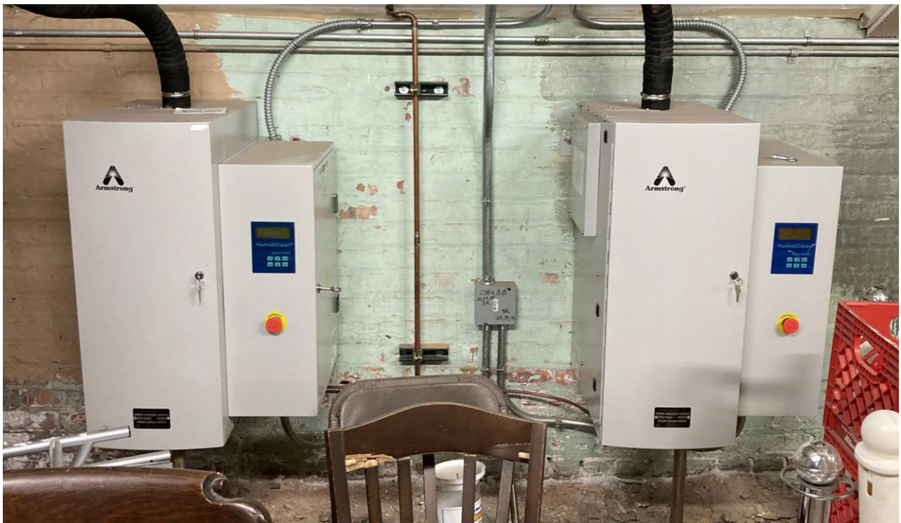
(UAC #1 and UAC #2-Existing Dehumidification Units)
