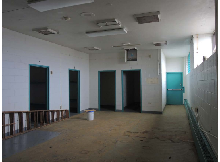
Photo 6: Block partition walls in areas of jail cells.
