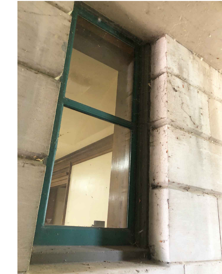
OBSERVATION: BOTH GREEN & GRAY WINDOW PAINT ARE PEELING & FADING RECOMMENDATION: SURFACE PREPARATION FOR MPI DSD 2 REMOVE & REPLACE DETERIORATED PERIMETER SEALANT
