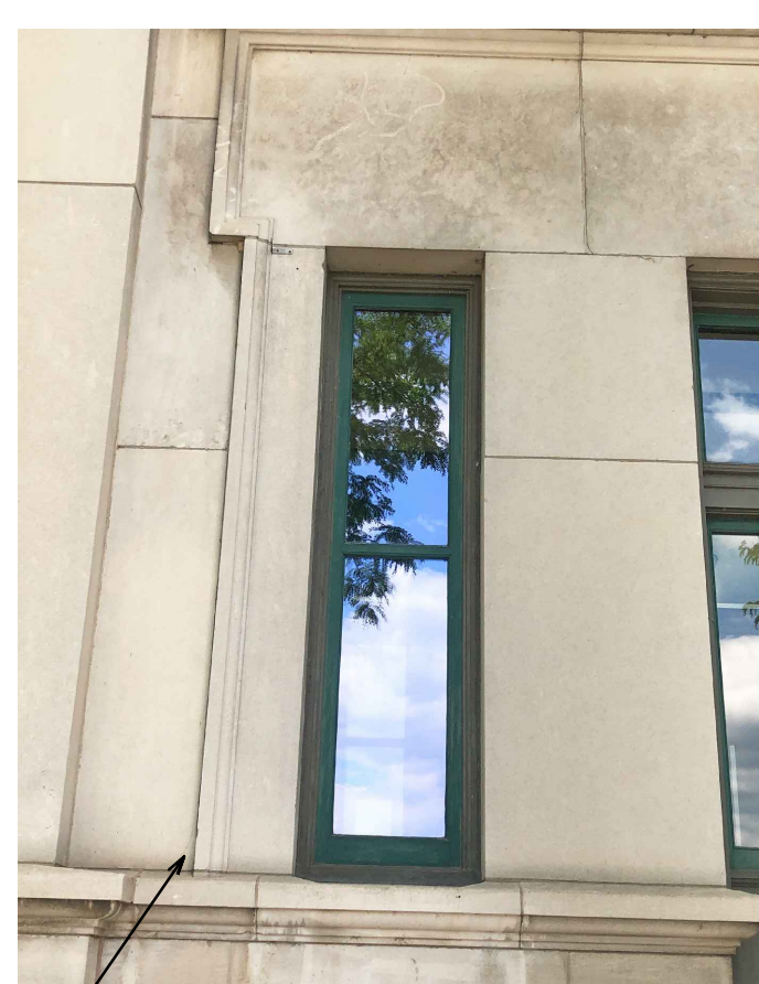
OBSERVATION: STONE UNIT IS CRACKED WITH NO APPARENT DISPLACEMENT. RECOMMENDATION: DETERMINE IF STONE IS LOOSE. IF CRACKED PIECE IS LOOSE, REPAIR BY SURFACE PATCHING. IF CRACKED PORTION IS SOUND, REPAIR CRACK.
