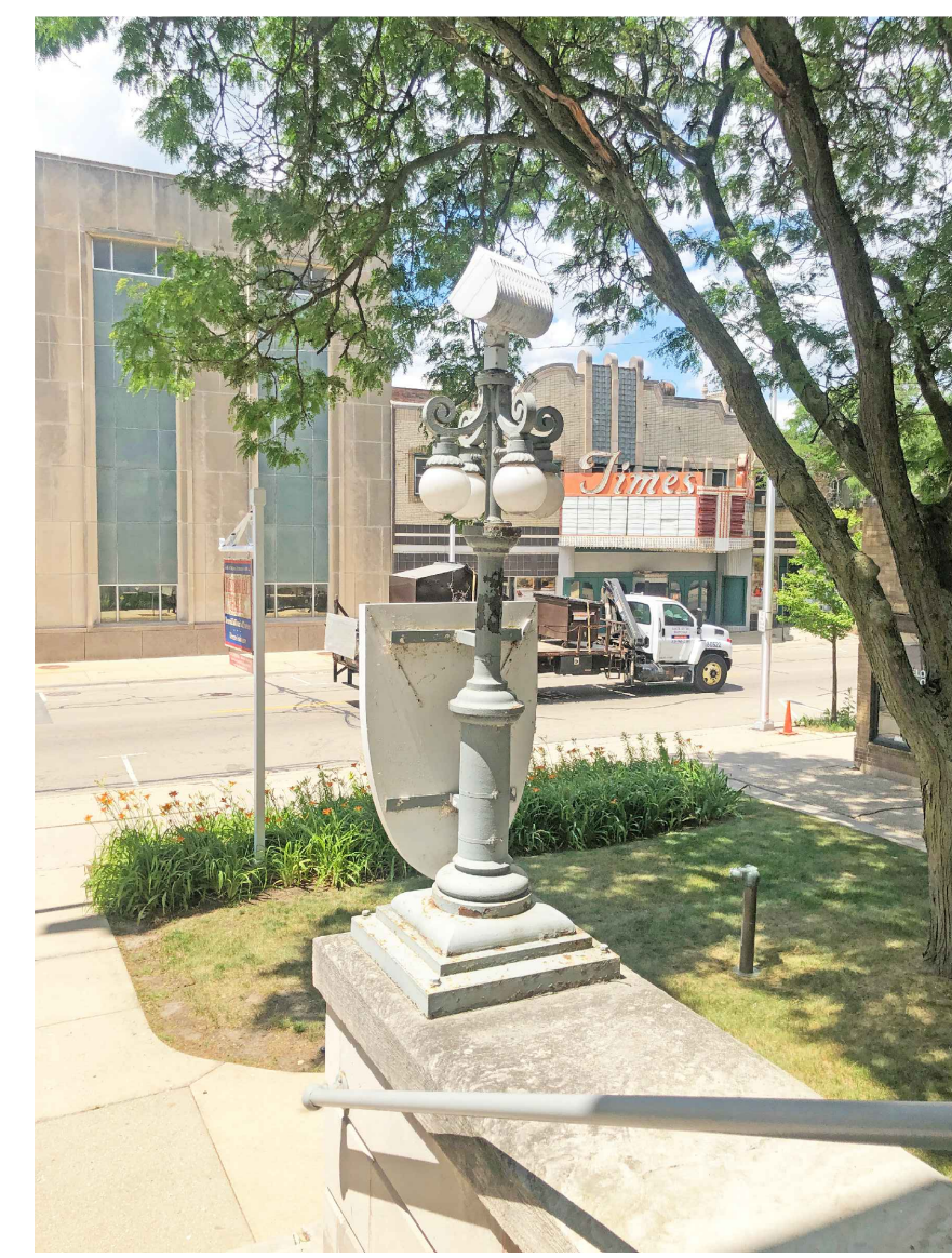
3 OBSERVATION: EXTERIOR STAIR LIGHT POSTS ARE SEVERELY RUSTED AND THE PAINT IS PEELING RECOMMENDATION: SURFACE PREPARATION FOR MPI DSD 3
