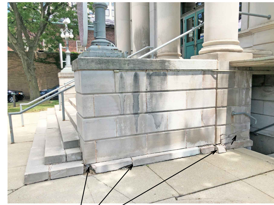
2 OBSERVATION: STONE BASE IS SEVERELY DAMAGED AND DISPLACED RECOMMENDATION: SEE STAIR WORK NOTES THIS SHEET
