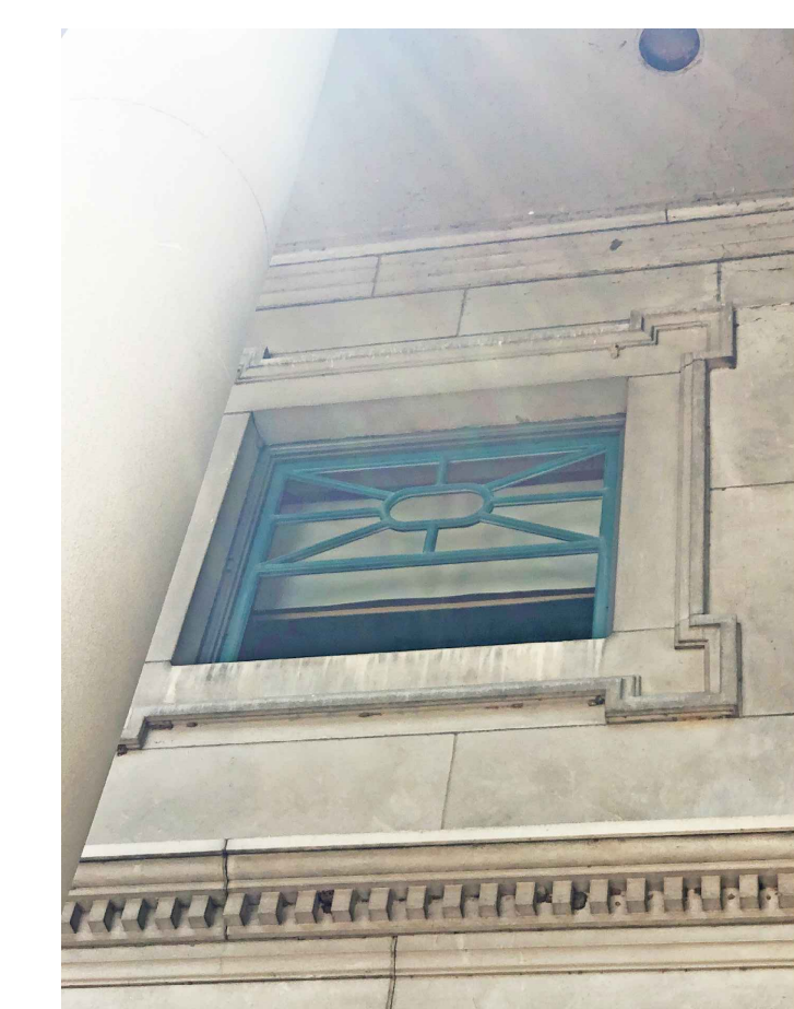
49 OBSERVATION: BOTH GREEN & GRAY WINDOW PAINT ARE PEELING & FADING. SOME WOOD DAMAGE OBSERVED. RECOMMENDATION: SURFACE PREPARATION FOR MPI DSD 4 REMOVE & REPLACE DETERIORATED PERIMETER SEALANT
