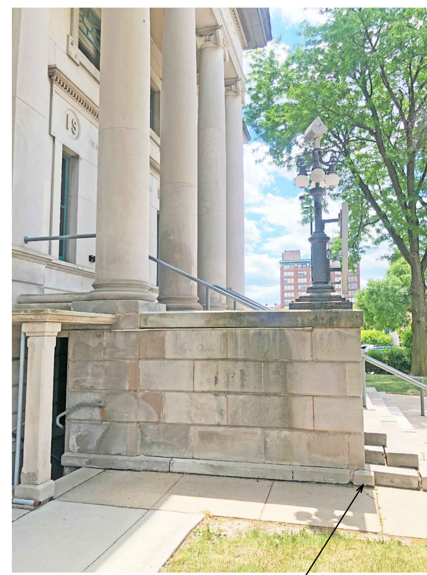
1 OBSERVATION: STONE CORNER IS SEVERELY DAMAGED AND DISPLACED RECOMMENDATION: SEE STAIR WORK NOTES THIS SHEET
