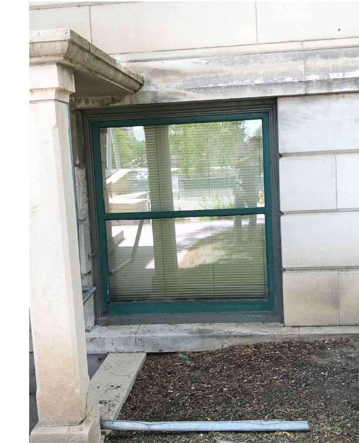
OBSERVATION: BOTH GREEN & GRAY WINDOW PAINT ARE PEELING & FADING RECOMMENDATION: SURFACE PREPARATION FOR MPI DSD 2 REMOVE & REPLACE DETERIORATED PERIMETER SEALANT
