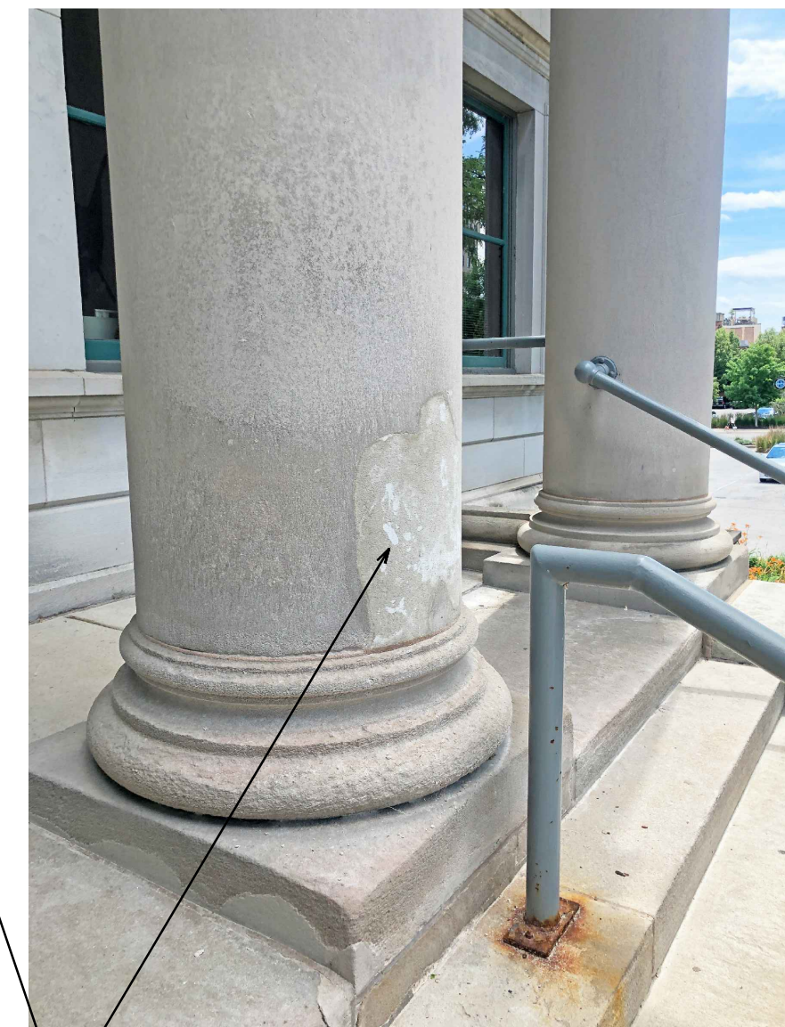
9 OBSERVATION: EXISTING STONE REPAIRS ON COLUMNS DON'T MATCH THE ORIGINAL STONE COLOR WELL RECOMMENDATION: CLEAN AND STAIN EXISTING REPAIR TO BETTER BLEND WITH THE ORIGINAL STONE
