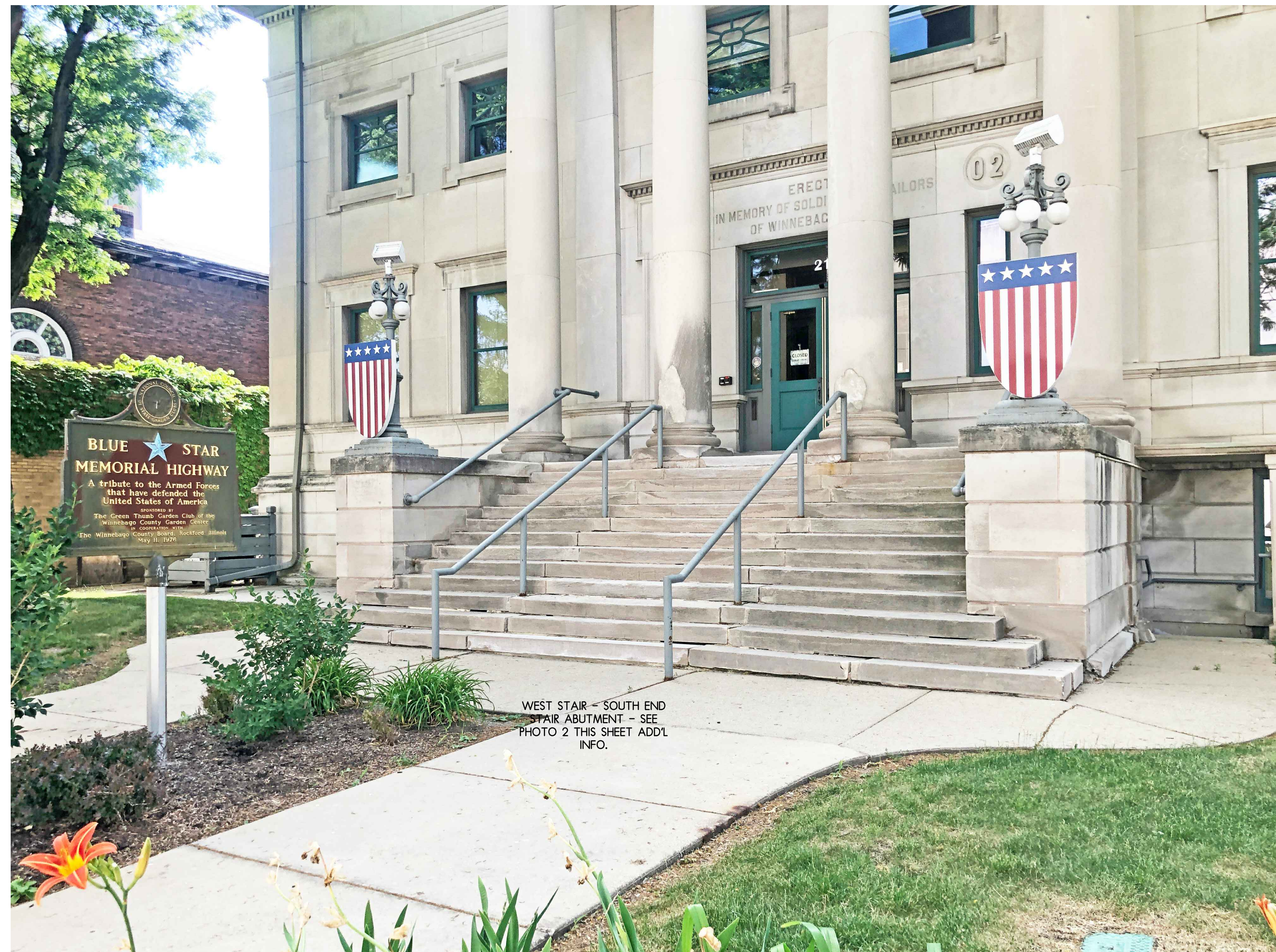
7 OBSERVATION: EXTERIOR STAIR HANDRAIL IS SEVERELY RUSTED AND THE PAINT IS PEELING RECOMMENDATION: SCRAPE AND REMOVE ALL LOOSE PAINT AND RUST, TREAT SOLID RUST, SAND OTHER SURFACES TO BLEND SURFACE FINISHES, CLEAN PRIME AND APPLY MIN 2 COATS FINISH PAINT.
