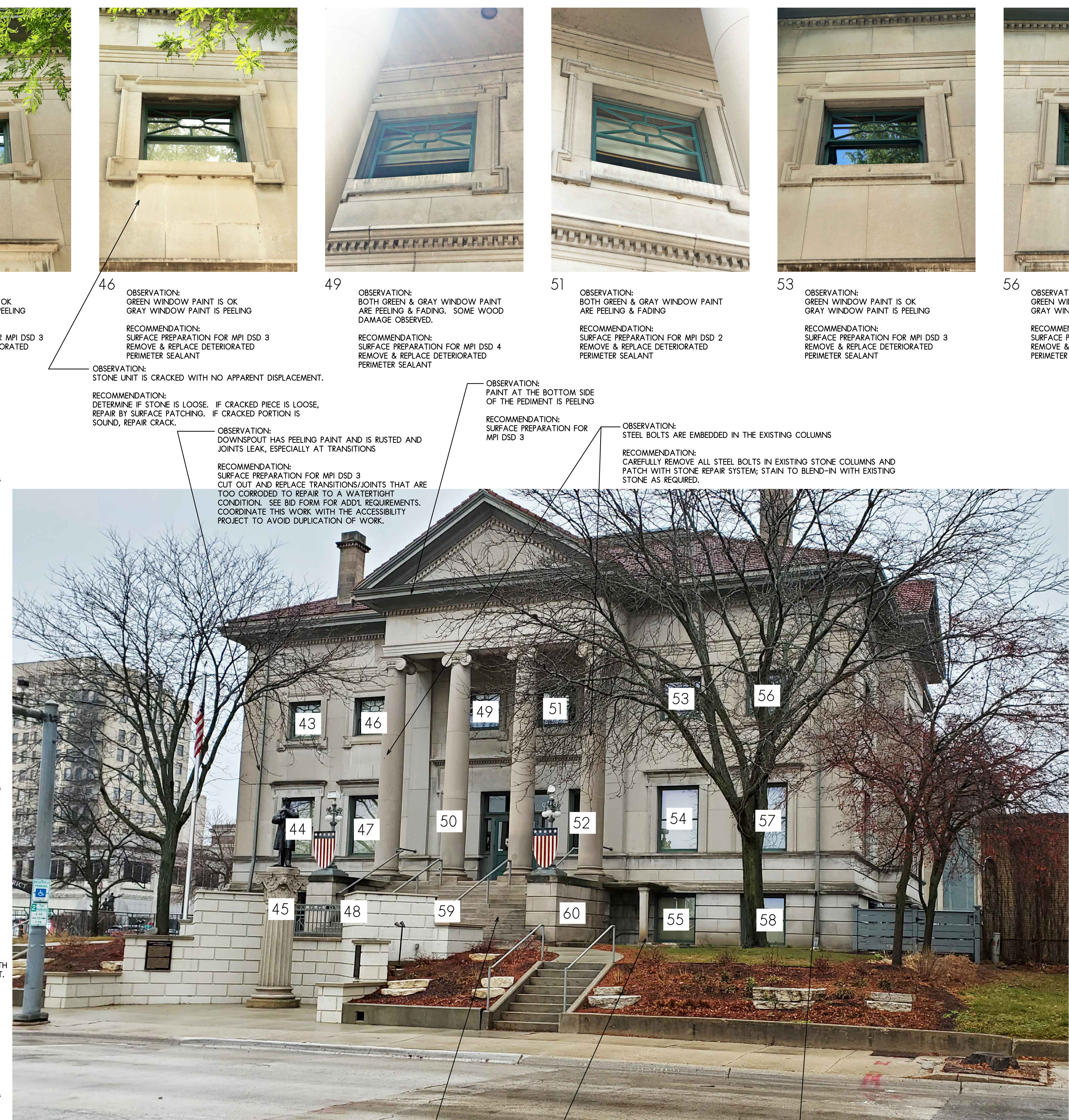
OBSERVATION: LIMESTONE COLUMN IS CRACKED AT THE BASE. RECOMMENDATION: DETERMINE IF STONE IS LOOSE. IF CRACKED PIECE IS LOOSE, REPAIR BY SURFACE PATCHING. IF CRACKED PORTION IS SOUND, REPAIR CRACK.
