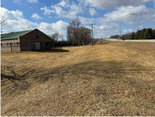
North Side of existing facility along highway
