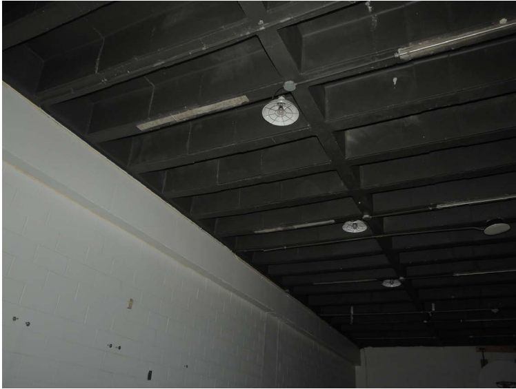
Photo 5: Reinforced concrete floor or roof supported along concrete block partition wall.
